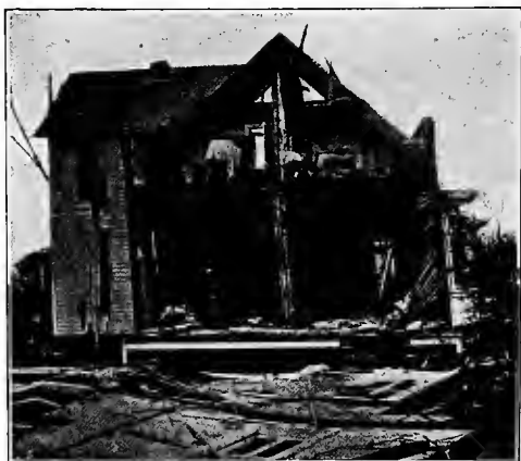
FIG. 474. — A house after one wall was blown out during a tornado.
